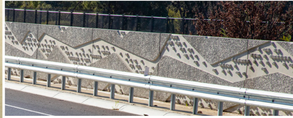
Photo: Imagine Pictures/Echuca-Moama Bridge Project
